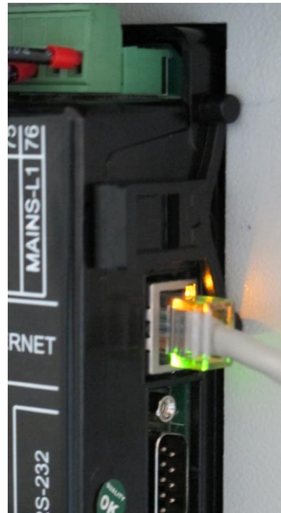
Installation of self-retaining type bracket
